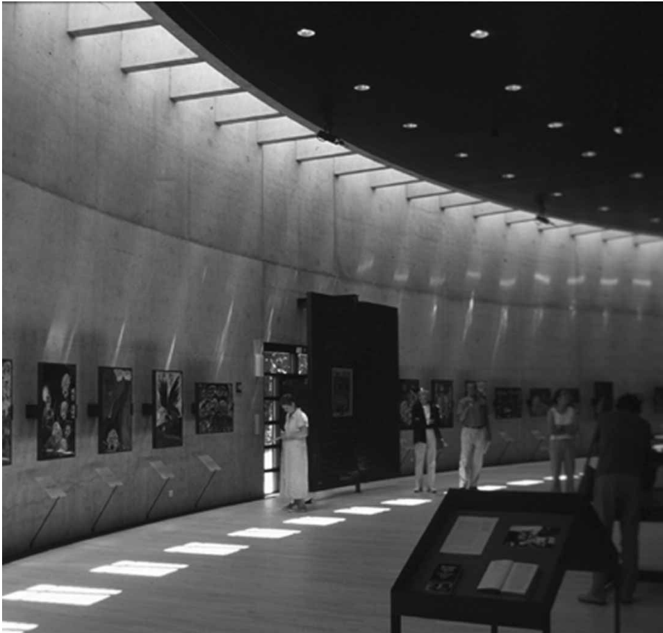
Figure 10. Under-ground exhibition hall illuminated by skylights on the terrace. (Source: author.)
